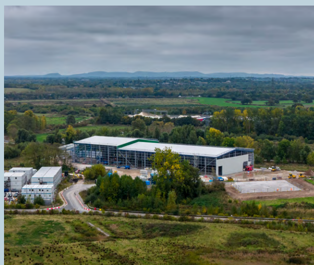
PET recycling plant in Ellesmere Port
