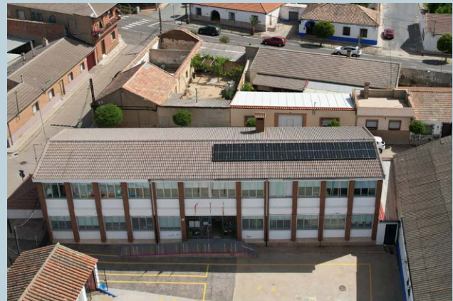
Successful PV installation at the school in Picón in January 2024
