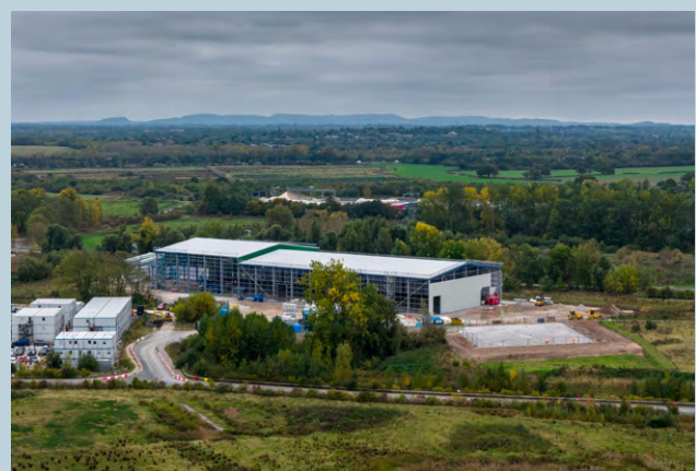
PET-Recyclinganlage in Ellesmere Port
